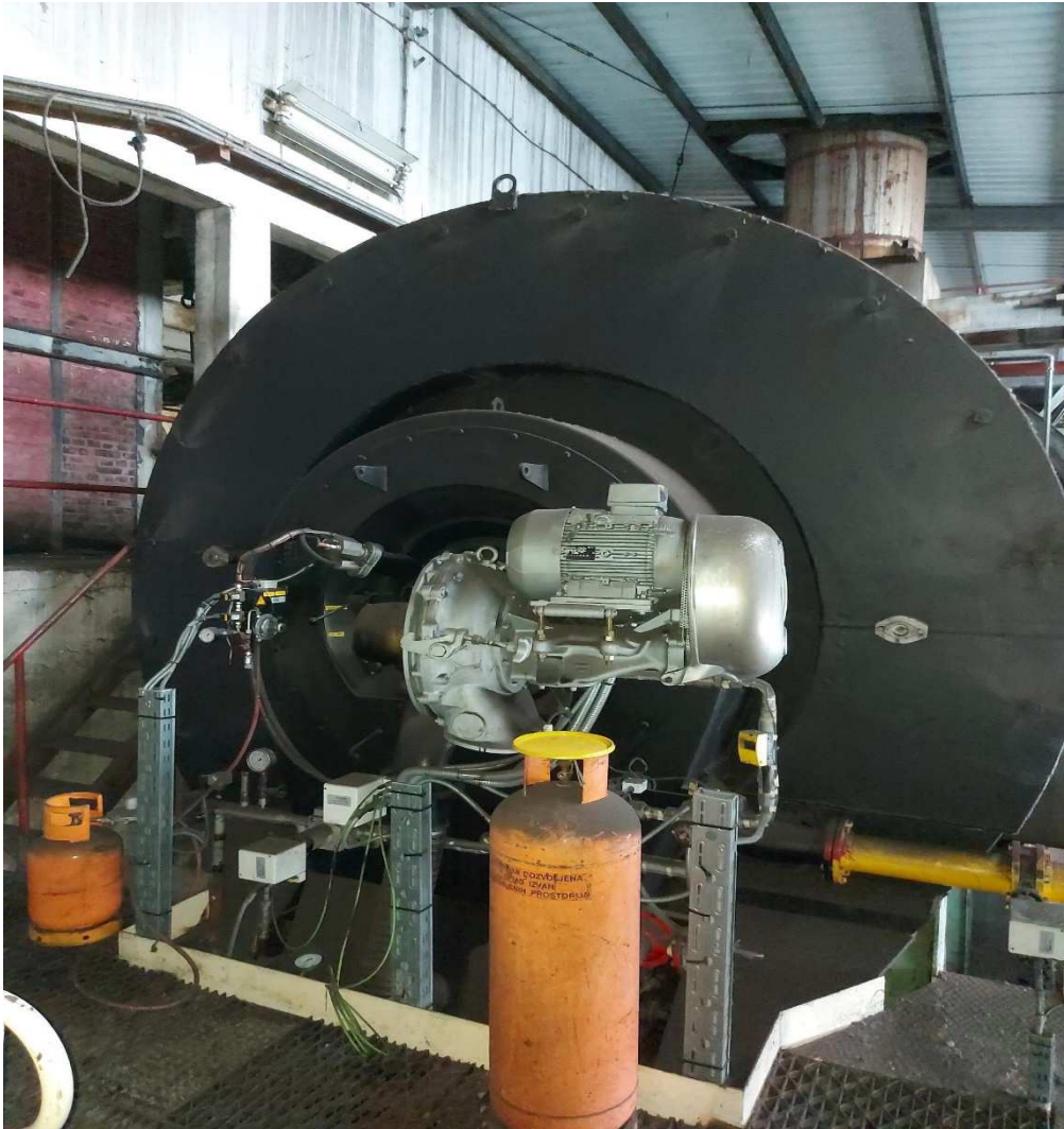
Combined gas/oil burner
